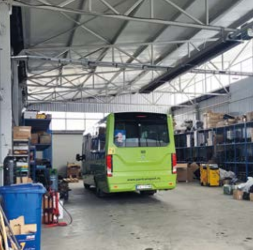
Bus hall for air-conditioning work on the vehicle.
